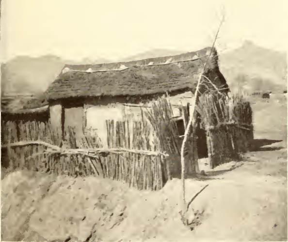
A TYPICAL NATIVE HUT, SHOWING FENCE MADE FROM STALKS OF "KAOLING" (TALL WHEAT), N. CHINA
