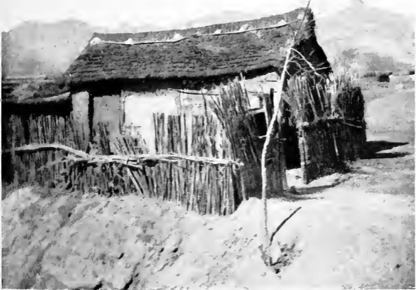
A TYPICAL NATIVE HUT, SHOWING FENCE MADE FROM STALKS OF "KAOLING" (TALL WHEAT), N. CHINA
