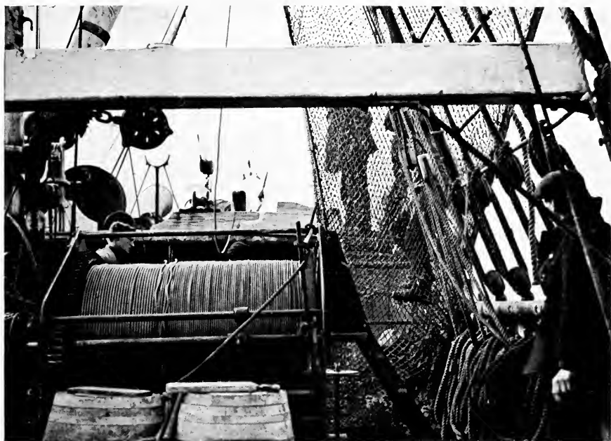
THE BIG WINDING-DRUM FOR THE DEEP-SEA DREDGING CABLE
