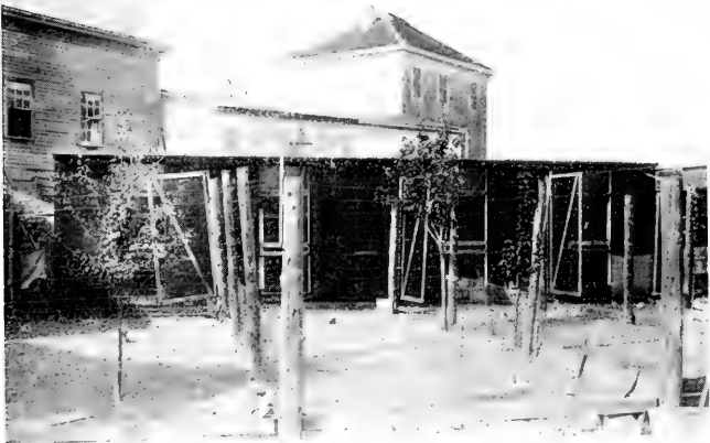
This house is made of building paper laid on poultry netting, without boarding
