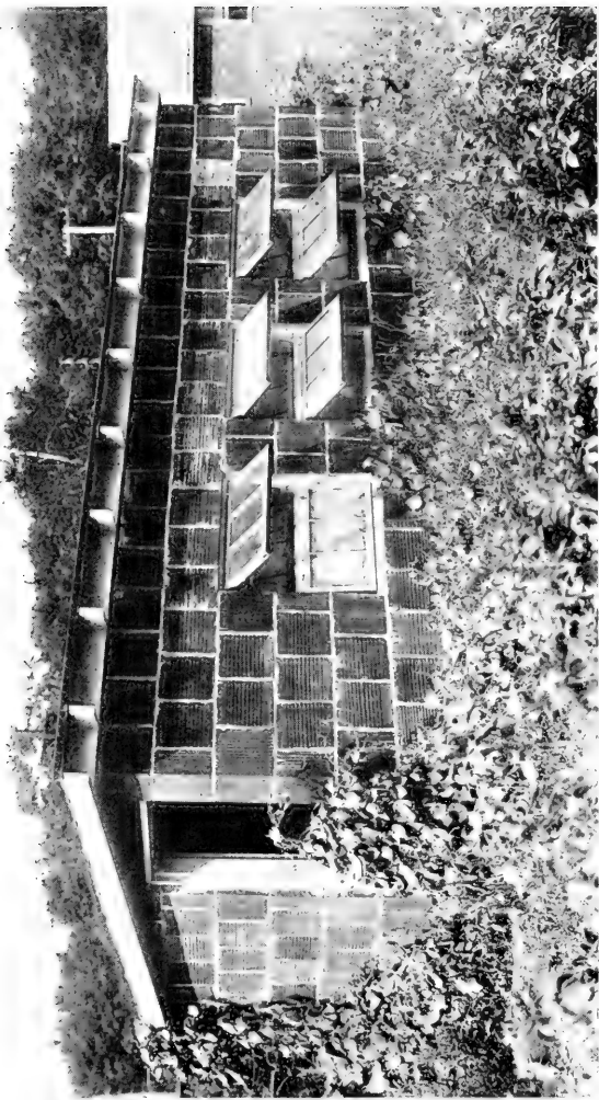
Incubator houses built of terra cotta hollow tile keep a very even temperature. The idea is a new one
