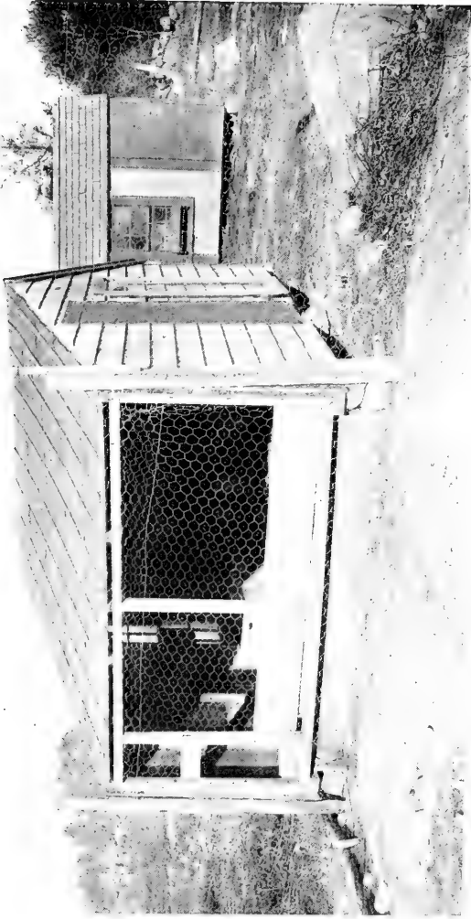
An example of the Tolman fresh-air house. The front is left open the year around, even in cold climates
