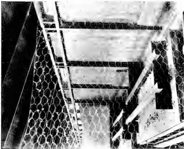
The openings, with shutters, at the back provide ventilation on hot nights
