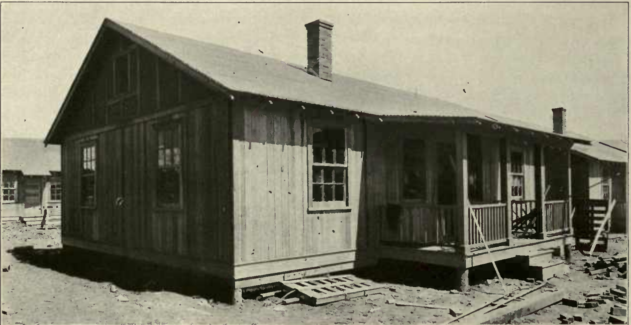
Sectional House Erected
