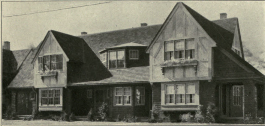
Three Family Cottage in the Housing Development at Derby, Conn., Built for Miss Frances E. Osborne. Murphy & Dana, Architects
