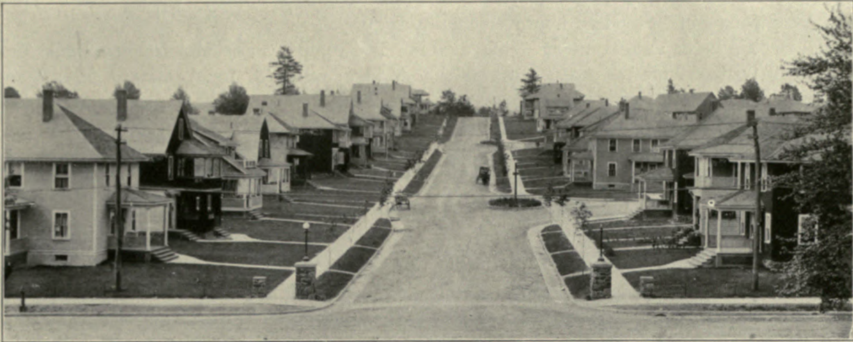
One hundred and two of these Houses were Erected in 102 Days at Endee Manor, Bristol, Conn.
