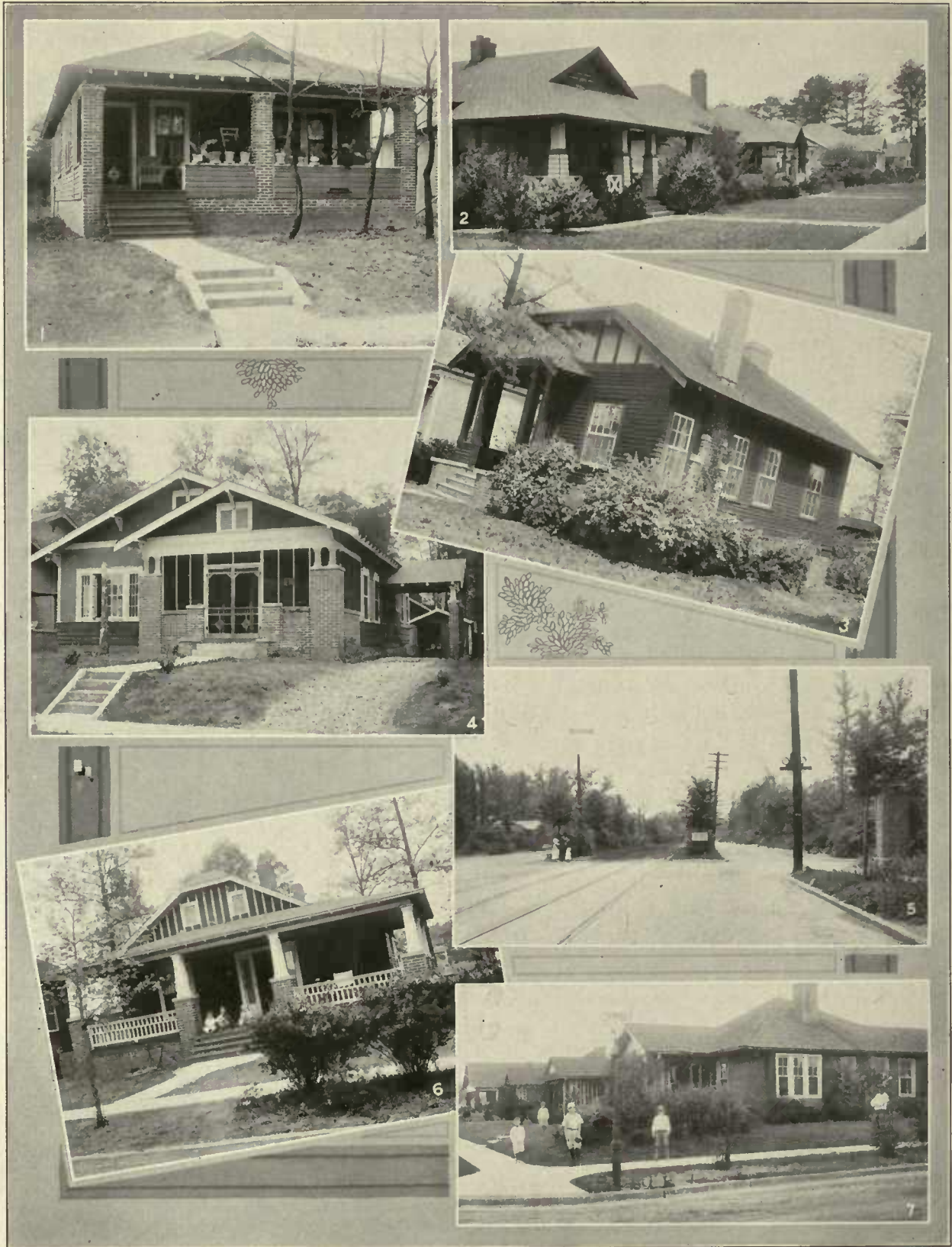
Entrance to Fairfield, and a Variety of Bungalow Types in that Model Development
