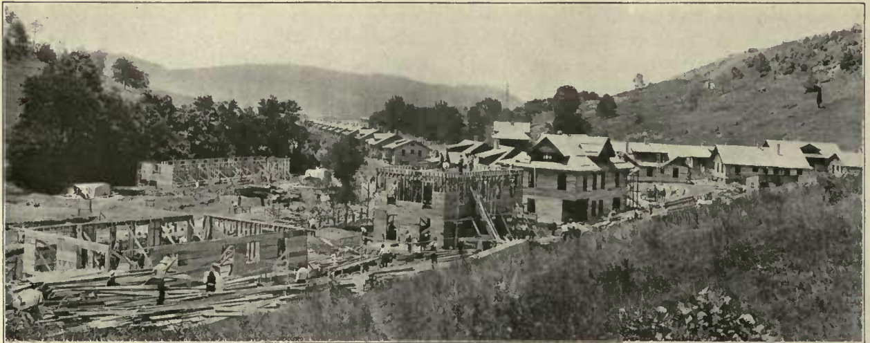
Area R.—Showing Houses Under Construction in Executive Residential Section
