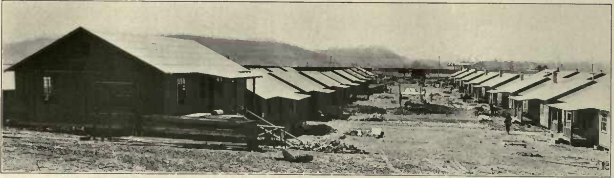
Street Showing Houses Completed
