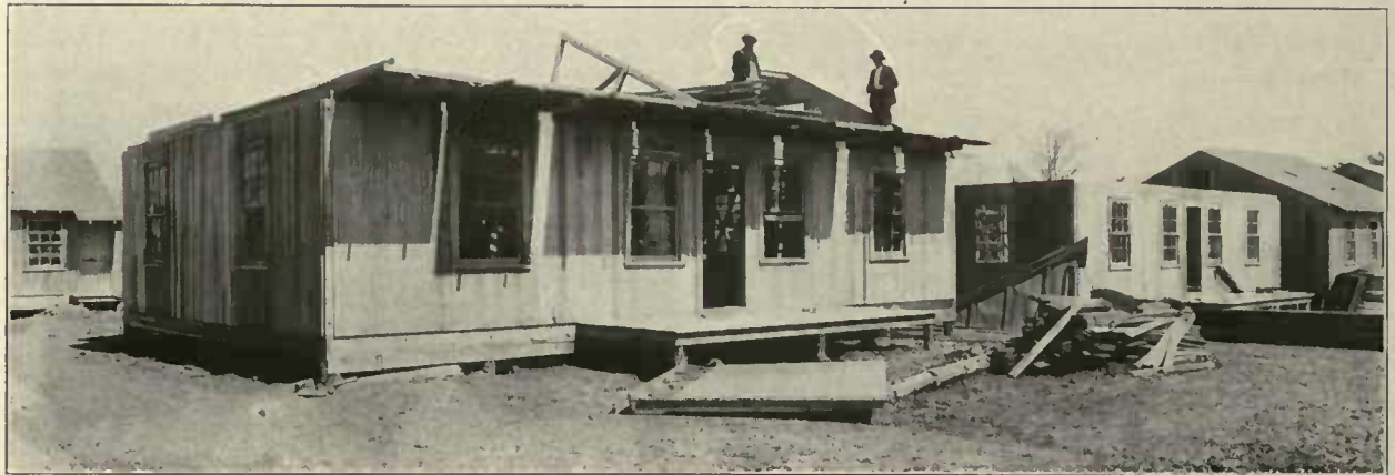
Walls Erected on Sectional Houses
