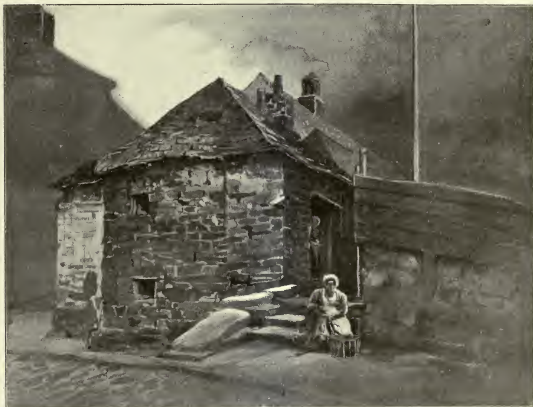
Cottage built on the Old City Wall, Plymouth.
