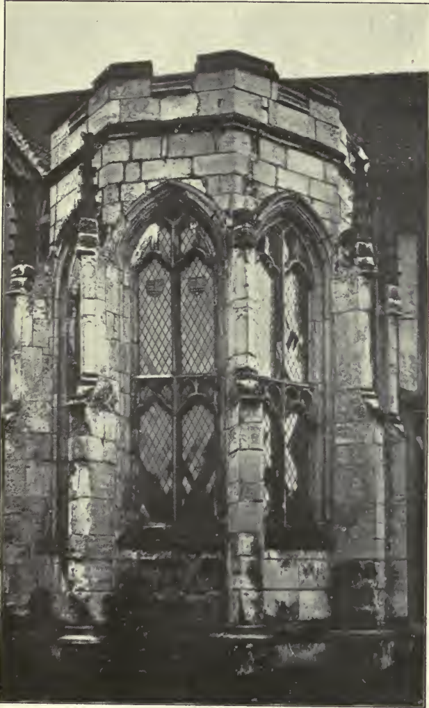
Oriel Window, Old Hall, Gainsborough.
