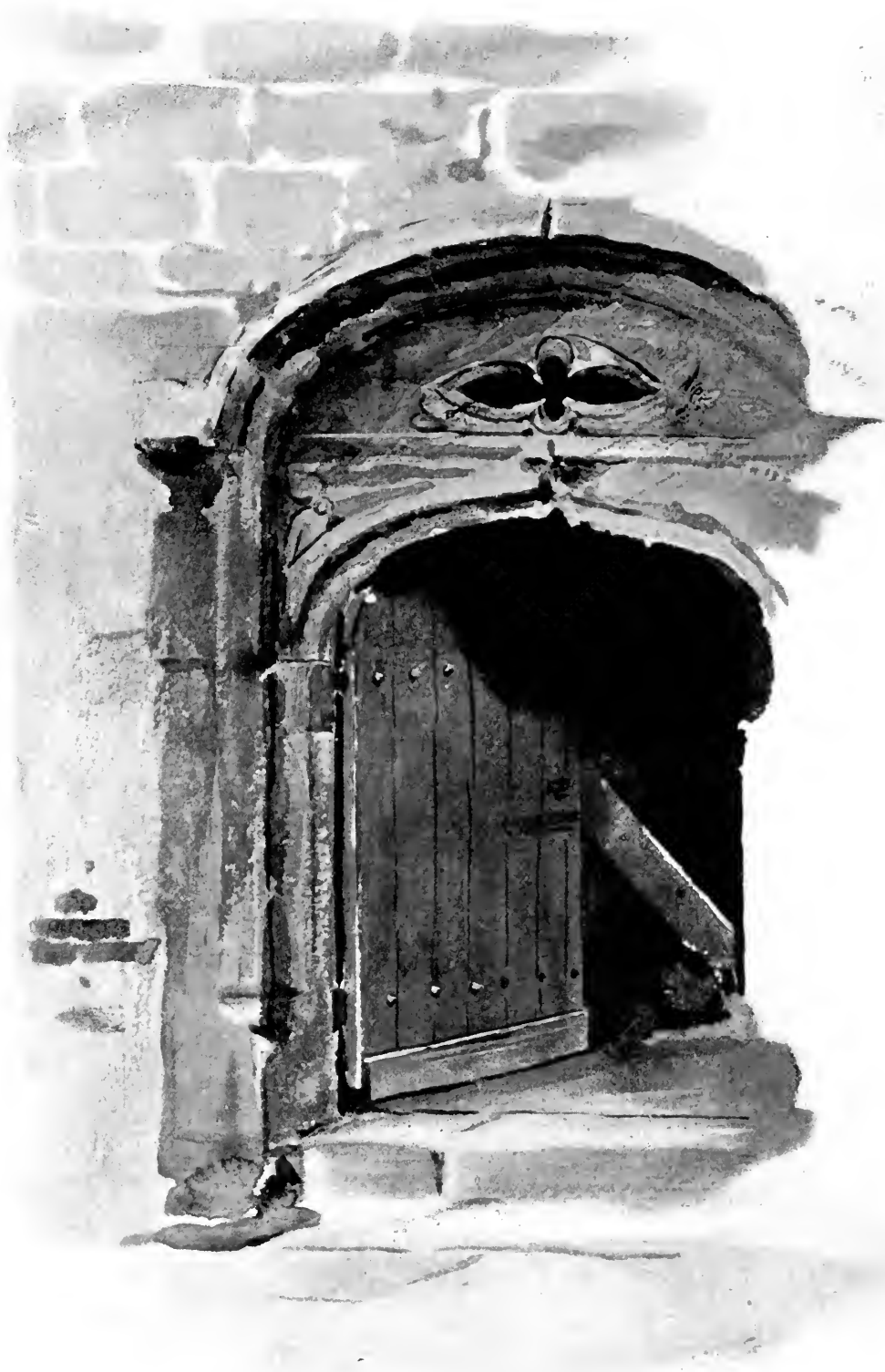
Doorway in the Priesten House, Plymouth.
