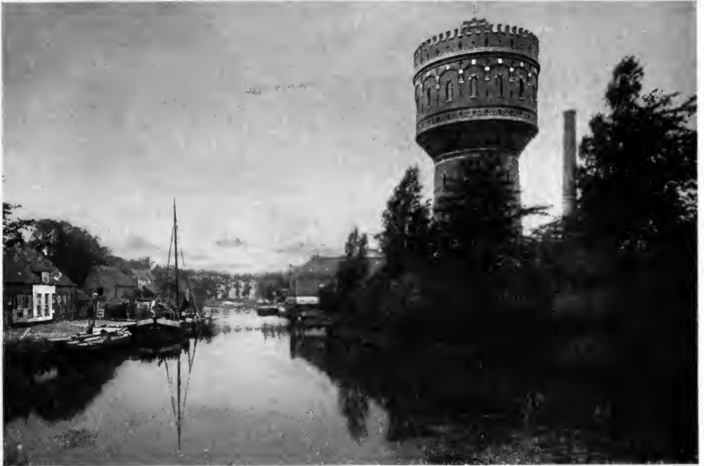
The Water Tower, Delft.
