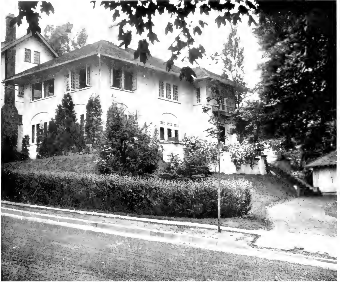
View from Road Side
