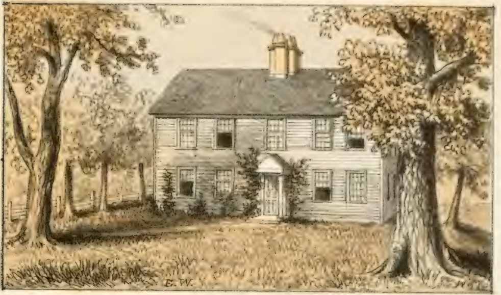
The Bradstreet House, North Andover.
