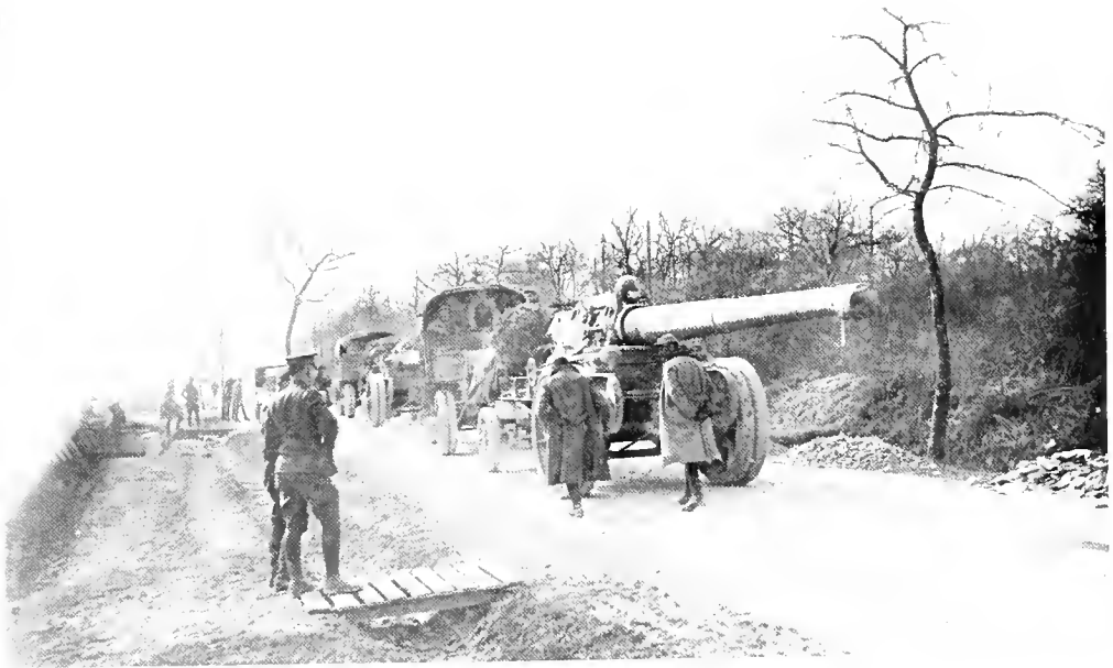
MOTORIZED APPARATUS ON THE WAY TO THE FRONT.
