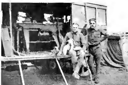
A Field Repair Station.
