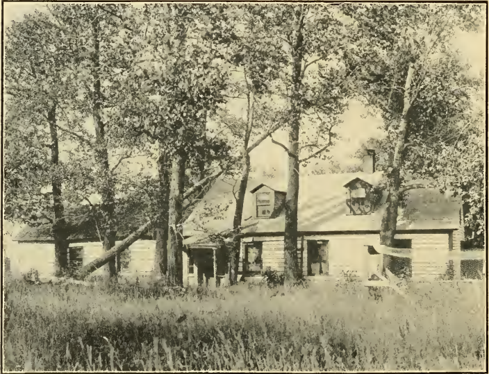
JOHNSTON'S HOUSE AS IT APPEARS TODAY—A VIEW FROM THE STREET FRONT.
