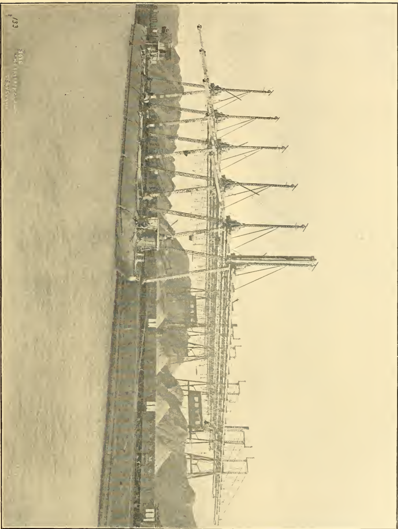
SHOWING THE THIRD STAGE OF ORE HANDLING—THE BROWN BRIDGE TRAMWAY. THESE MACHINES WERE OPERATED BY STEAM POWER
