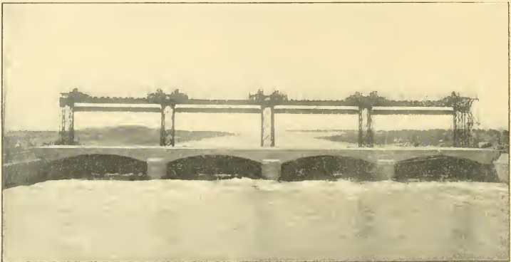
HEAD GATES, POWER CANAL, MICHIGAN, LAKE SUPERIOR POWER CO.
