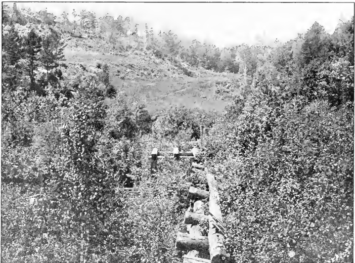
THE SITE OF THE OLD JACKSON FORGE ON THE CARP RIVER, NEAR NEGAUNEE, SHOWING REMAINS OF OLD DAM FORGE, BUILT IN 1847-48.
