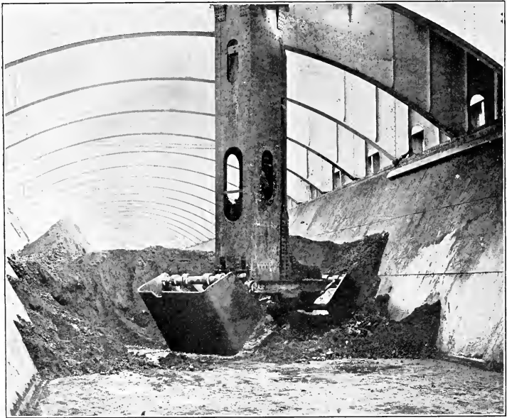
THE HULETT CLAM-SHELL BUCKET IN THE WOLVIN'S HOLD.
