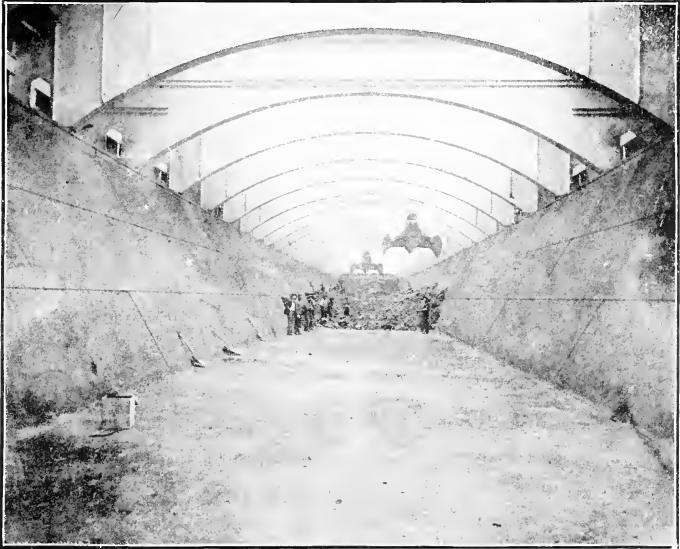
THE BROWN GRAB BUCKET IN THE HOLD OF THE STEAMER WOLVIN.
