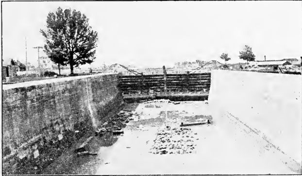
ORIGINAL UPPER LOCK OF 1855.
