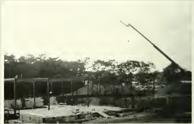
and now the start of our new building
