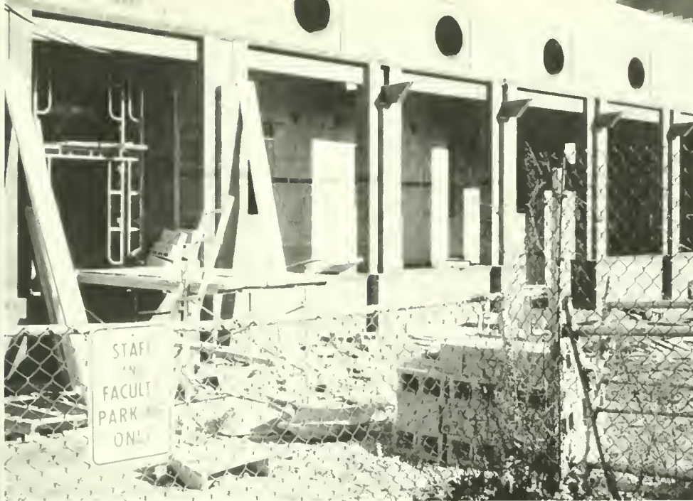
construction going on here . . . .
