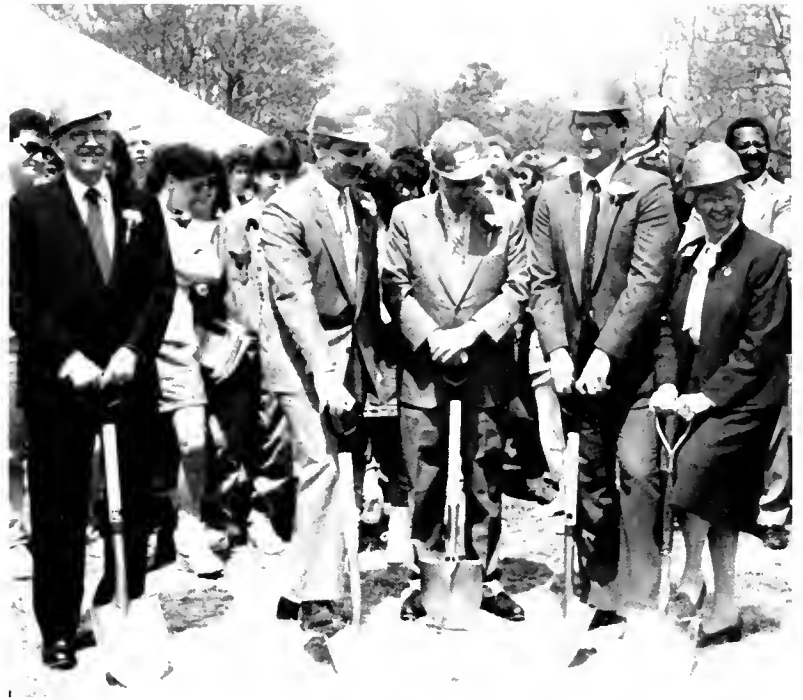
Ground breaking - spring semester '88
