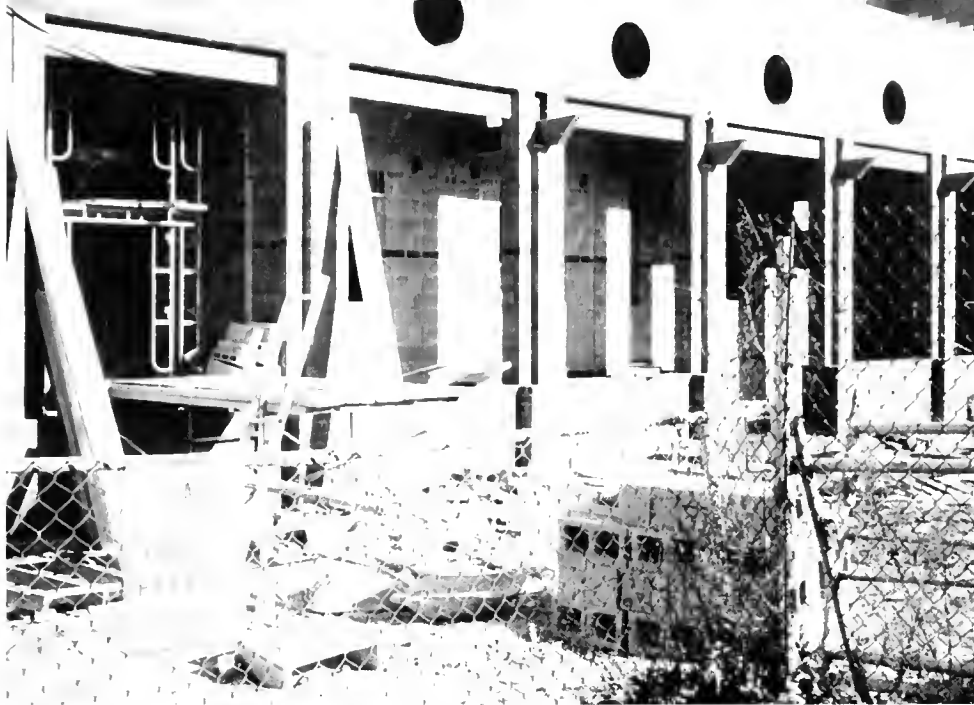
construction going on here . . . .
