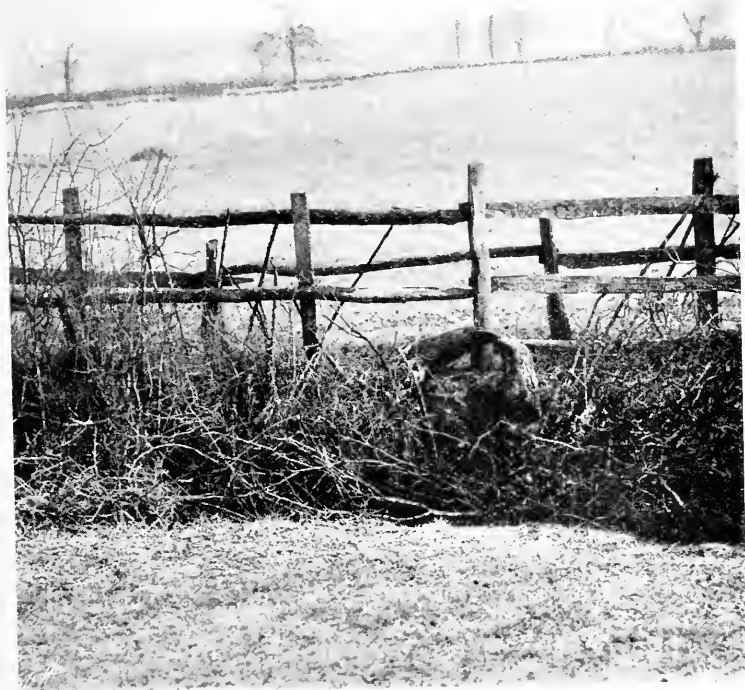
Fig. 111.—Posts and rails with ditch.
