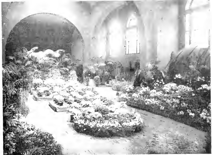
GENERAL VIEW OF PART OF MAIN HALL.
