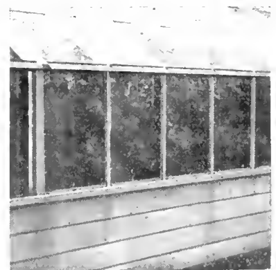
At the eye, the Patented Ice-Protecting plate, with sash bar clasp attached, is used.
