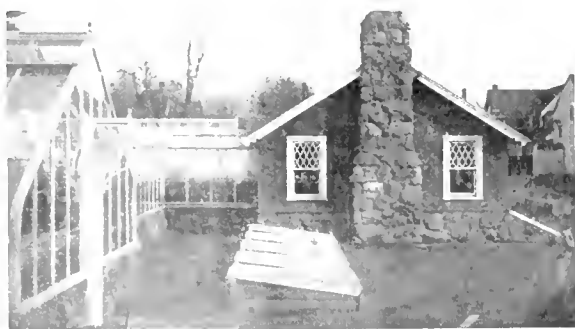
By connecting the potting-house by a 11 feet passage the shading of the central house is overcome and valuable space for propagating benches secured.
