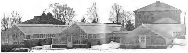
New Greenhouses and Instruction Building for Floriculture and Market Gardening at Massachusetts Agricultural College.
