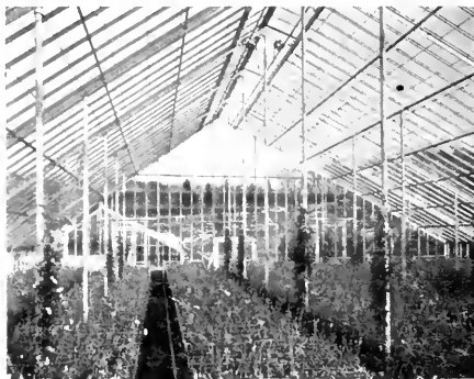
Interior, looking towards same gable.
