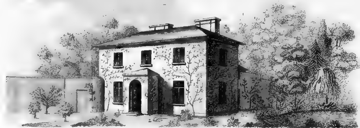
View of the Gardeners House
