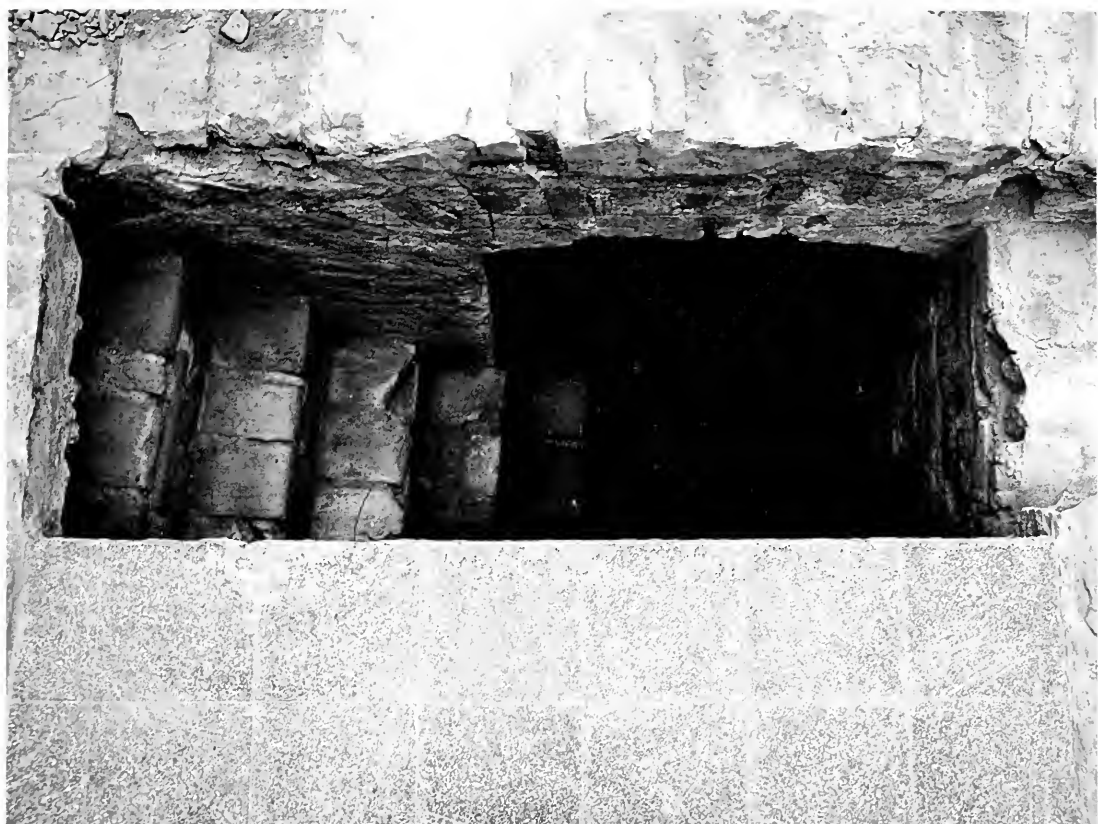
FIG. 19. Our excavations revealed an L-shaped stairway leading into and down to the 2.50-m-long entrance.
