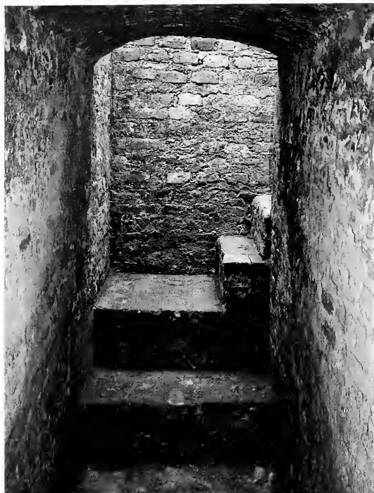
FIG. 20. The entranceway to the vaulted structure.
