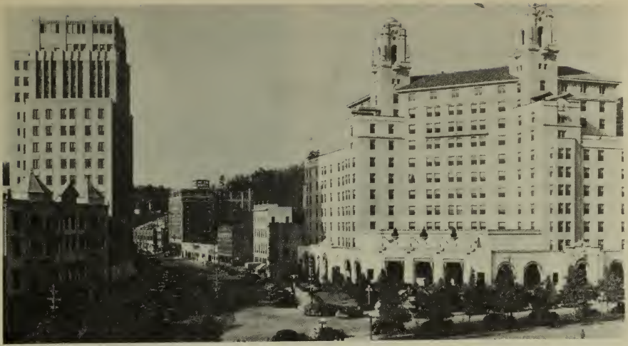
CENTRAL AVENUE, CITY OF HOT SPRINGS
