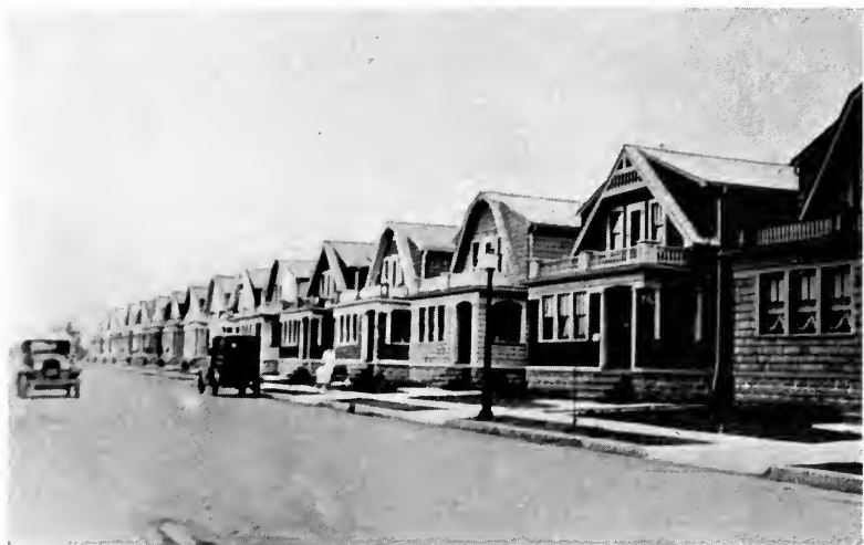
An example of the undesirable repetition of a single type of Buffalo house on a series of too narrow lots.
