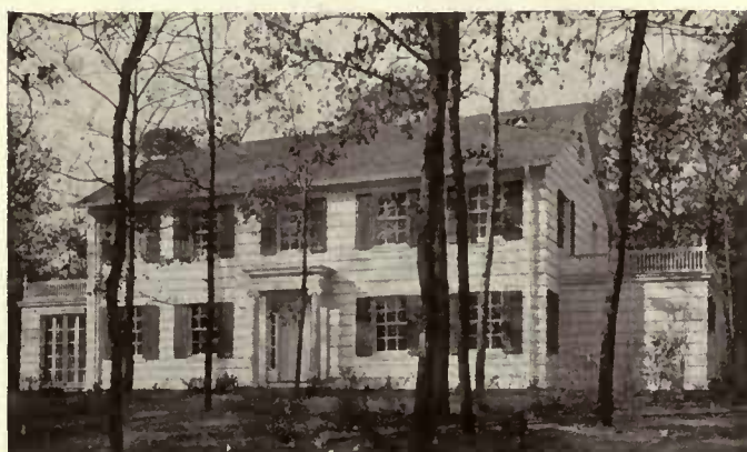
House of George McBride, Esq., Highland Park, Ill. Robert F. Seyfarth, Architect, Chicago, Ill.
