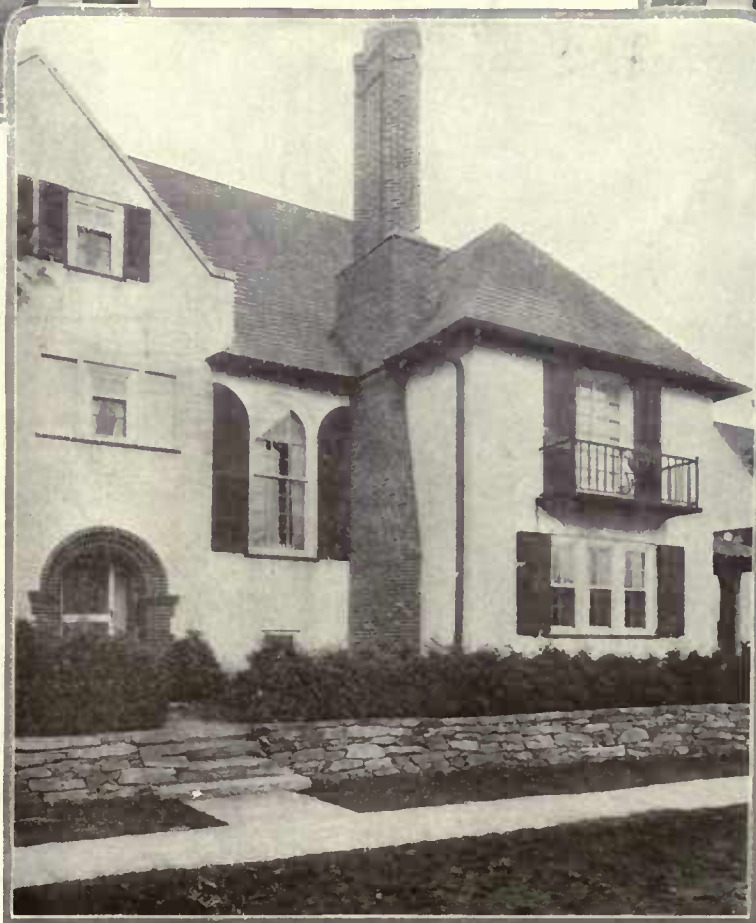
In planning a façade the architect deals with spaces and voids—spaces the wall, voids the windows, and upon the juxtaposition of the two depends his success. In this house, of which Edmund B. Gilchrist is architect, several types are shown—round-top stairs window, a French window with balcony, double hung sash windows alone and in pairs, and in one instance, flanked with panels later to be filled with Della Robbia plaques
