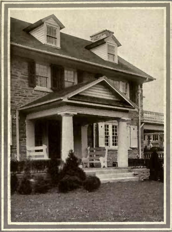
The sturdy type of Doric column. While the column itself reveals an adherence to precedent, the frieze which it supports is an adaptation, reflecting the present day tendency to simplicity
