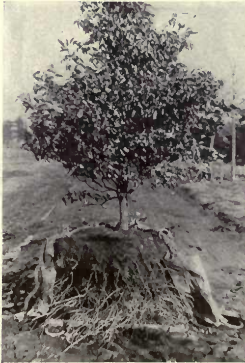
With small trees the root system is carefully dissected and both roots and soil tied in a burlap container
