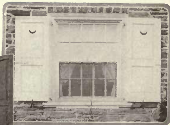
The Pennsylvania Colonial type of window in which shape, panes and shutters are the three elements. The shutter hardware is a local style capable of adaptation
