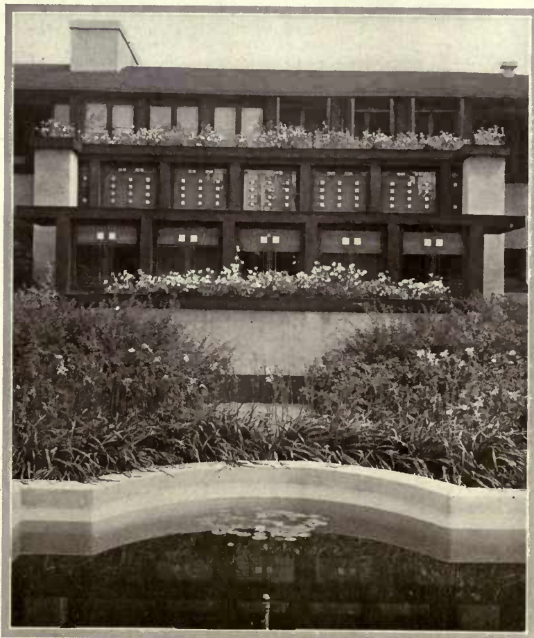
The residence of E. E. Boynton, Esq., at Rochester, N. Y., is built along the Frank Lloyd Wright lines, admitting an unusual display of window-boxes. Pitkin & Weinrichter, landscape architects
