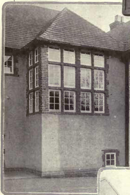
If the nature of the rest of the façade permits, staircase windows are unquestionably the most interesting for the architect and housebuilder. Varied uses and positions allow numerous forms. An unusual treatment in this house, designed by Edmund B. Gilchrist, is the tiered and brick mullioned staircase corner casement window above
