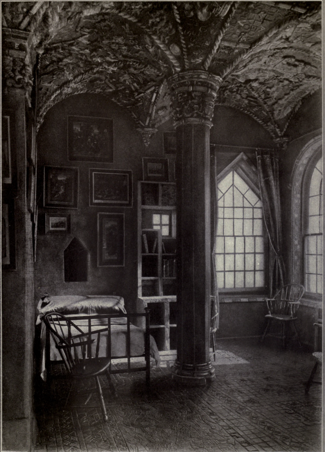
The infinite uses of cement and tile for interior finish and decoration, and even for built-in fittings, are graphically shown in "Font Hill," the residence of Charles Chapman Mercer, Esq., at Doylestown, Pennsylvania. The Columbus Room, one of the numerous bedrooms, boasts a tessellated tile floor and arched tile ceiling that give the feeling of real Italia
