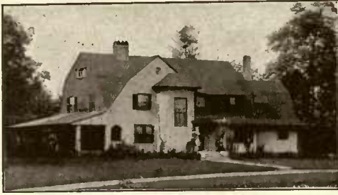
Stained with Cabot's Creosote Stains Karl Scott Putnam, Architect, Northampton, Mass.
