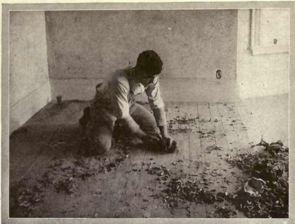
Hard-wood floors require a level sub-floor. They should not be laid until the plastering is thoroughly dry and all the other woodwork in the room finished
