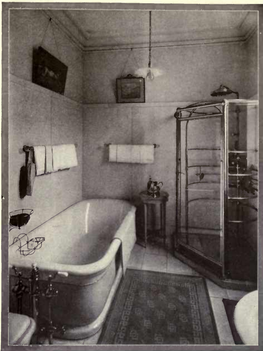
Figure V—No matter how elegantly fitted, the modern bathroom is incomplete without a modern shower. In this room the shower is entirely enclosed in glass with nickeled frame, the base receptor of solid marble
