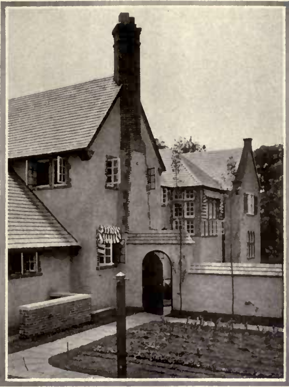
In this country house, of which Edmund B. Gilchrist is architect, brick trim has been attractively combined with rough concrete finish
