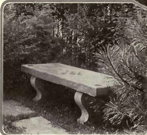
The ingenious gardener can make his own seat out of concrete. This type requires a very simple mould. Tiles are let into the top slab
