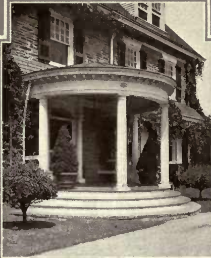
To be successful, the semi-circular porch must have a wide approach on either side. Here it is used with a Pennsylvania type of Colonial architecture
