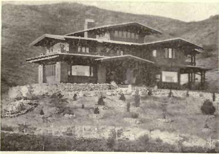
Courtesy of the Architectural Record A Pacific Coast type—a residence at Los Angeles, California E. B. Rust, architect
