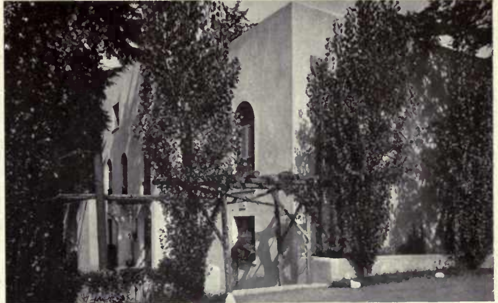
Hollow tile was used—6,500 of them put in place by three masons and seven helpers in twenty-seven working days. The whole was then covered with cement. There is one chimney to serve the four flues
