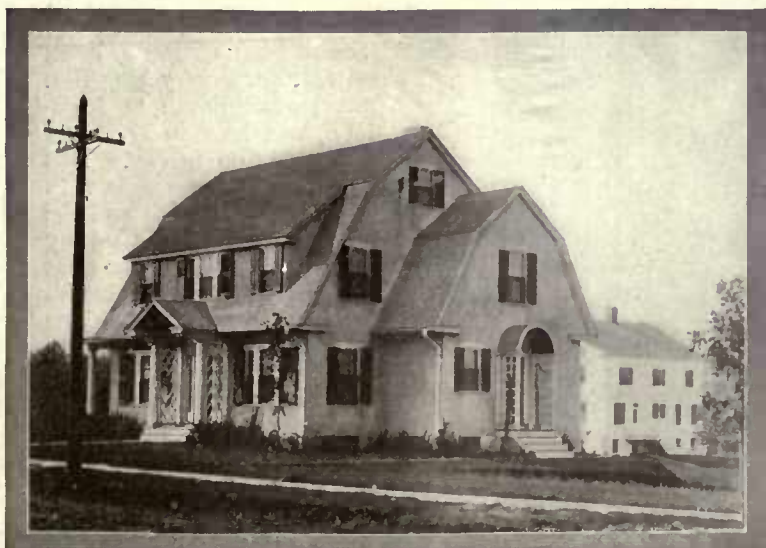
A. Raymond Ellis, architect This one, built of frame, stucco and shingle in Hartford, Conn., cost $6,500. The difference is due to materials
