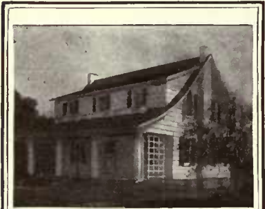
Stained with Cabot's Creosote Stains C. M. Hart, Architect, Bay Shore, N. Y.
