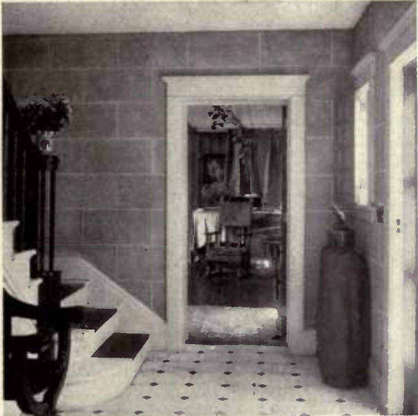
The vestibule walls are soft brown, the plaster laid directly on hollow tile. The marble floor is from an old dismantled house
