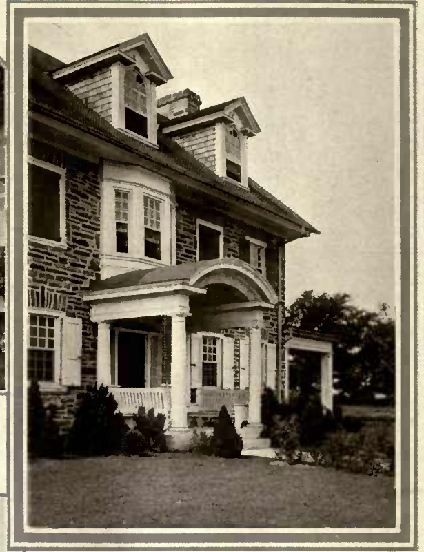
The Roman Doric column has been used here. Its characteristic is its proportion—the height being eight times the diameter, thus assuring, under usual conditions, a graceful appearance
