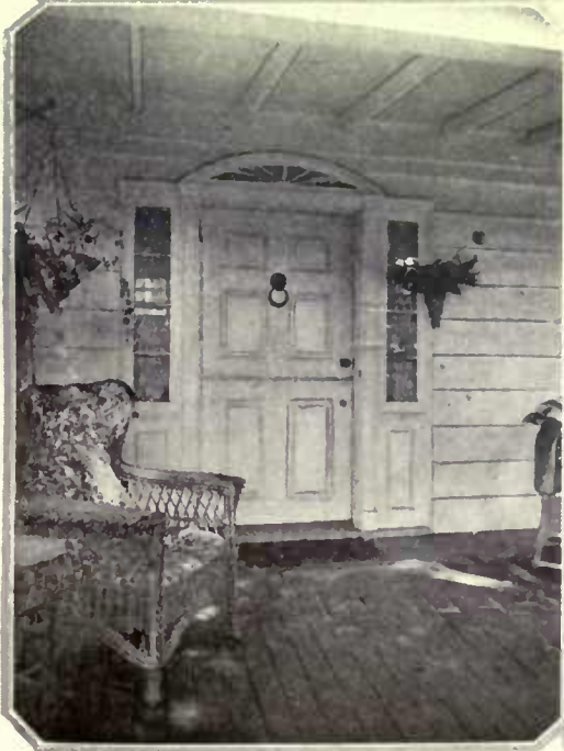
The new Dutch door was especially designed for the house. The shallow fan light is in proportion with the low ceiling of the porch
