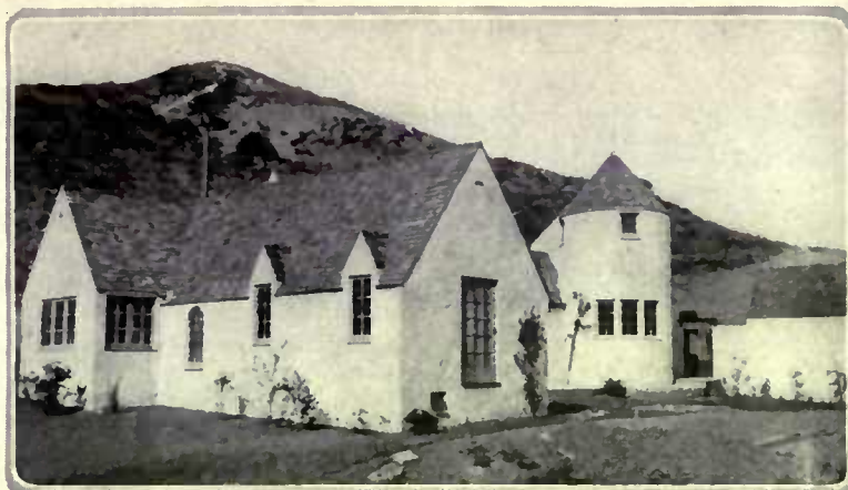
Near Hollywood is a one-story cottage reminiscent of the French farmhouse. At one corner rises a round tower, with maid's room above and dining room below
