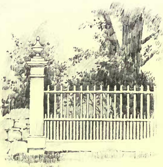
In the State of Massachusetts this dignified and white-painted fence with its simple cornerpost
