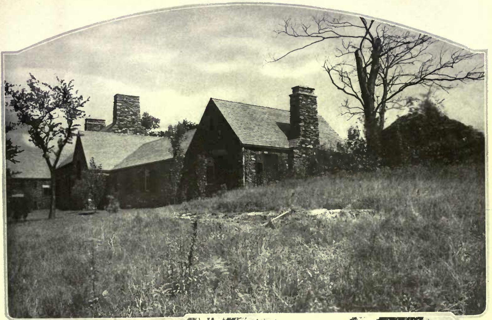
The house is set in a field and the natural effect preserved. Gables break the slate roof much in the way that rocks crop up through the soil
