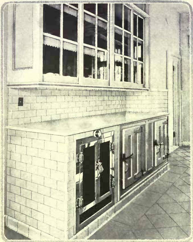
The plate warmer and refrigerator are in non-interfering proximity under the steel shelves of this kitchen dresser. C. P. H. Gilbert, architect. Bramhall, Deane Co.
