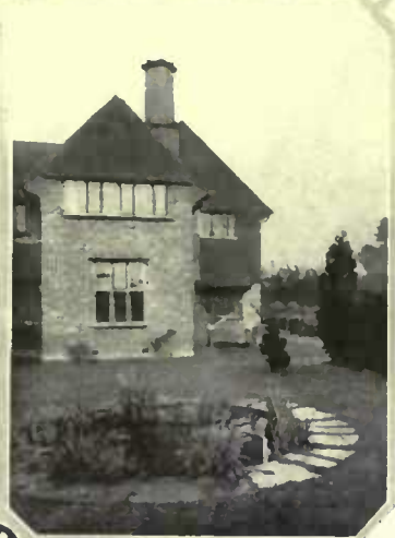
The library bay window looks out on this little pool and stretch of lawn. The pool's rim, as are the garden paths, is made of flagstones laid in the turf
