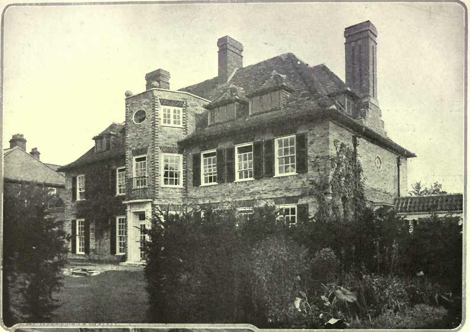
The west, or garden front opens on to a large lawn surrounded by tall planting. All the windows on the first floor extend to the ground. Their white trim and green shutters contrast pleasantly with the tawny, irregular color of the brick
