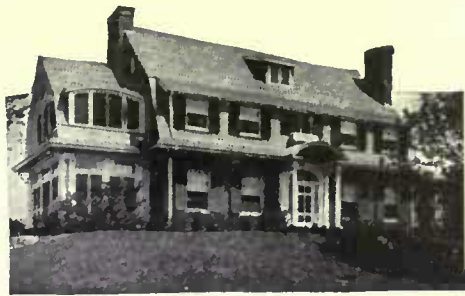
Equipped with Kernerator Residence of W. F. Wallace, Winnetka, Ill. Architects: Brown & Wolcott
