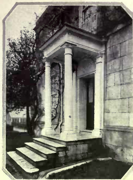
The severe simplicity of the front façade is broken by a classical portico with a white plaster fan device over the door
