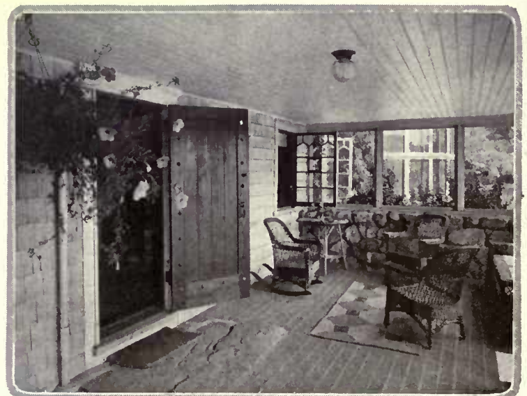
The sun porch is an all-year place, with a fieldstone foundation and sliding glass doors above. Wicker has been used and fibre mats
