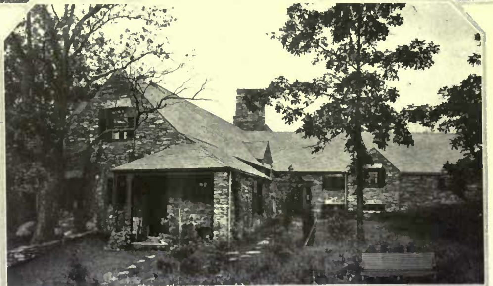
The servants' end and back porch are on one level and the owner's studio above them on the second. A guest door to the terrace is beyond
