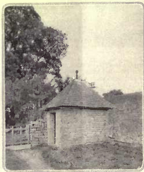
At The Court, Broadway, is a little Cotswold type of building, an excellent termination to strengthen the appearance of the garden wall. It is designed to keep garden tools
