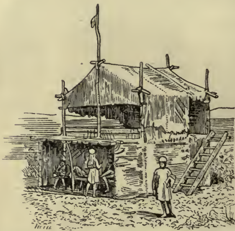
TWO-STORIED TENT COVERED WITH SKINS
