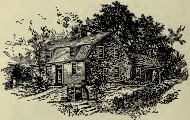
Rhode Island and Connecticut Shore House, with Gambrel Roof and "L" From "Homes in City and Country"
