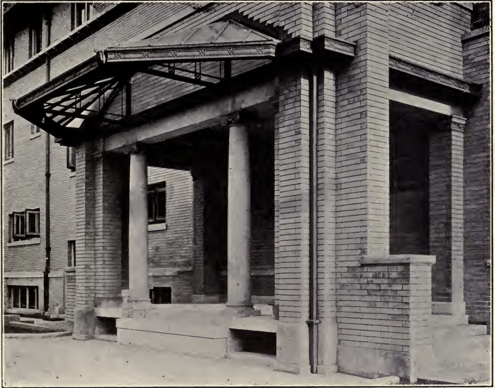
A WESTERN ENTRANCE
