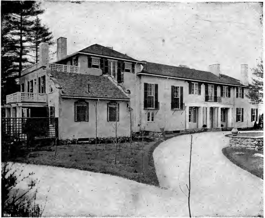
DOORWAY AND APPROACH
