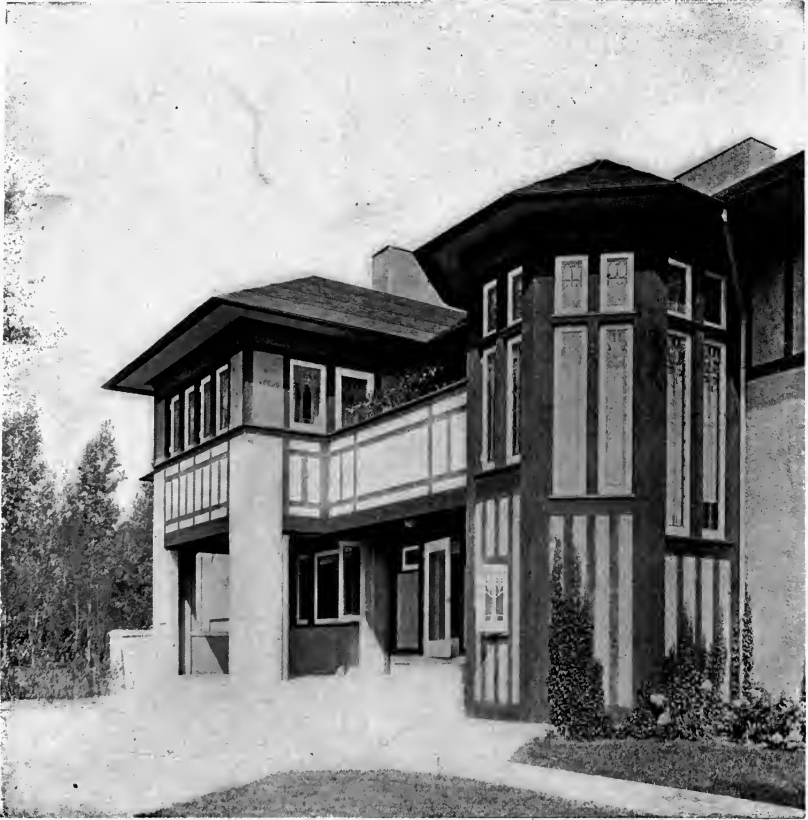
A SIMPLE TREATMENT OF BRICK AND PLASTER
