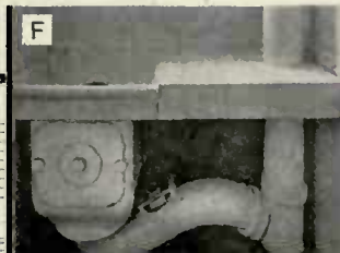
F. Garchey garbage remover. G. Hood over unit heater.
