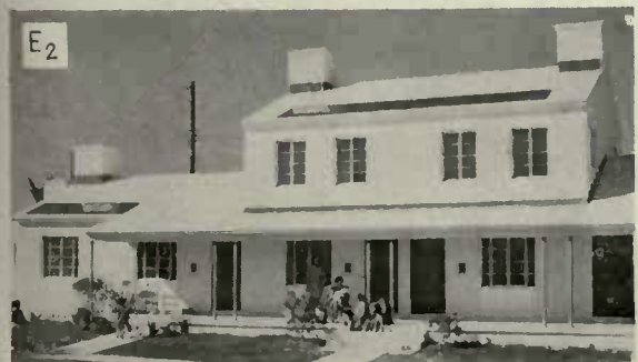
E. Miami, Fla. Edison Courts. Coverage 18.4%, density 40. Black patches on roof are glass covered solar heating units for hot water heating; the hot water tanks take the form of chimneys. Arch'ts. H. D. Stewart et al.
