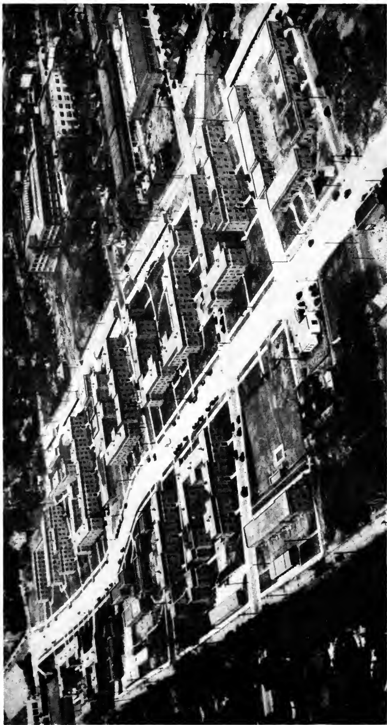
TECHWOOD HOUSING PROJECT, ATLANTA, GEORGIA. A W.P.A. ENTERPRISE.
