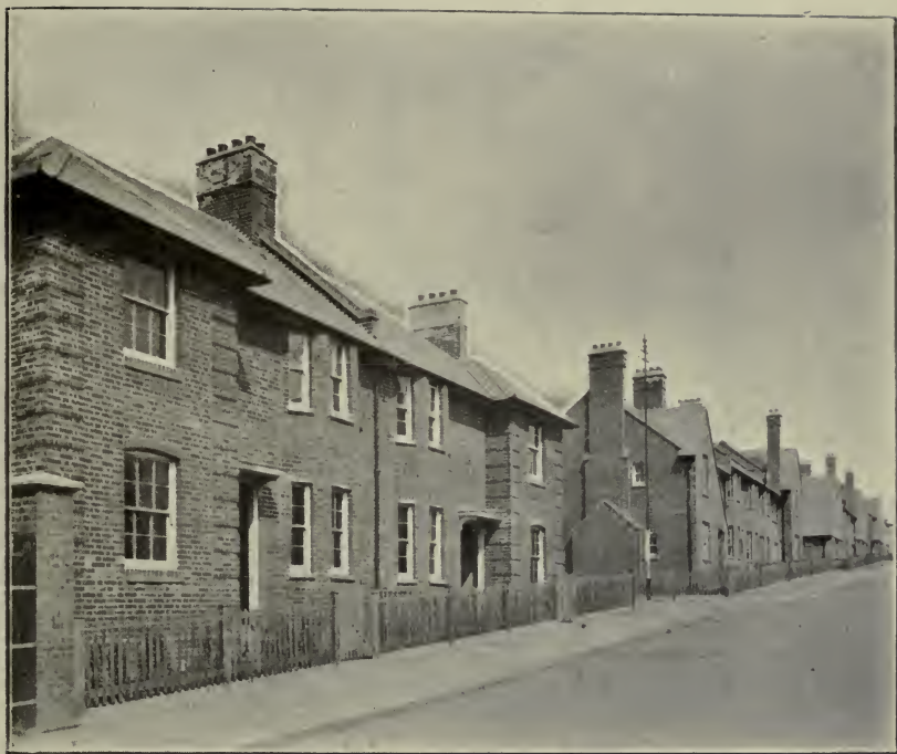
TOTTERDOWN FIELDS ESTATE—OKEBURN ROAD (WEST SIDE).
