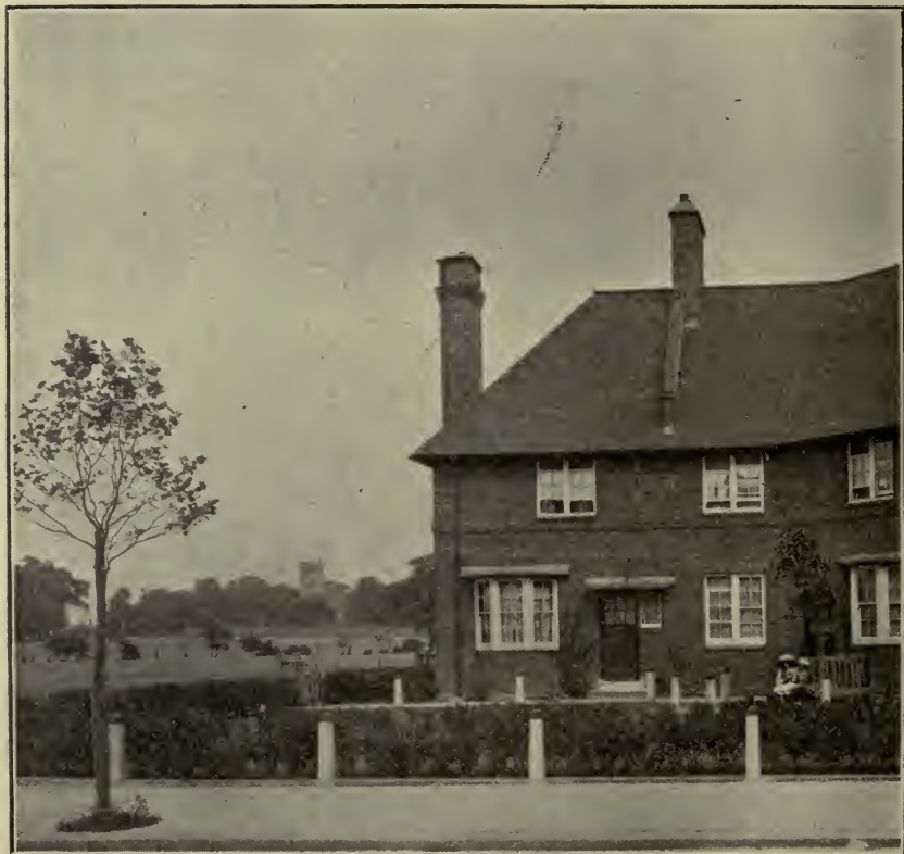
WHITE HART LANE ESTATE—CORNER OF AWLFIELD AVENUE (EAST ANGLE BLOCK).
