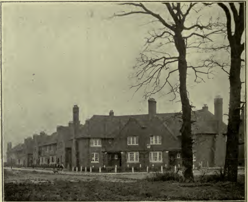
WHITE HART LANE ESTATE—AWLFIELD AVENUE (WEST ANGLE BLOCK).
