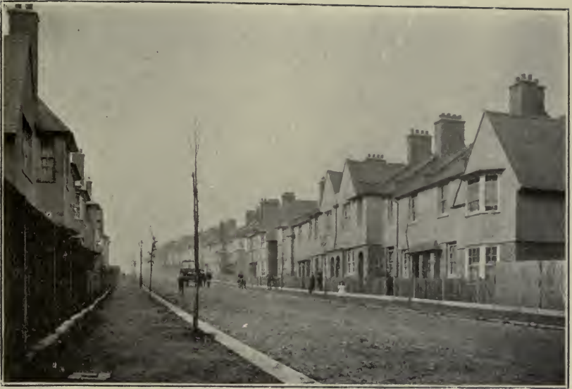
NORBURY ESTATE—TYLECROFT ROAD (LOOKING WEST).
