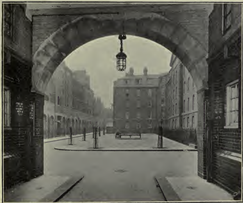
UNION BUILDINGS ESTATE.—LANEY BUILDINGS AND KIRKEBY BUILDINGS.
