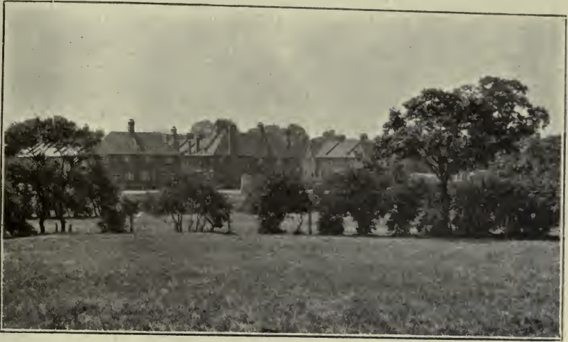
WHITE HART LANE ESTATE—GENERAL VIEW FROM NORTH.
