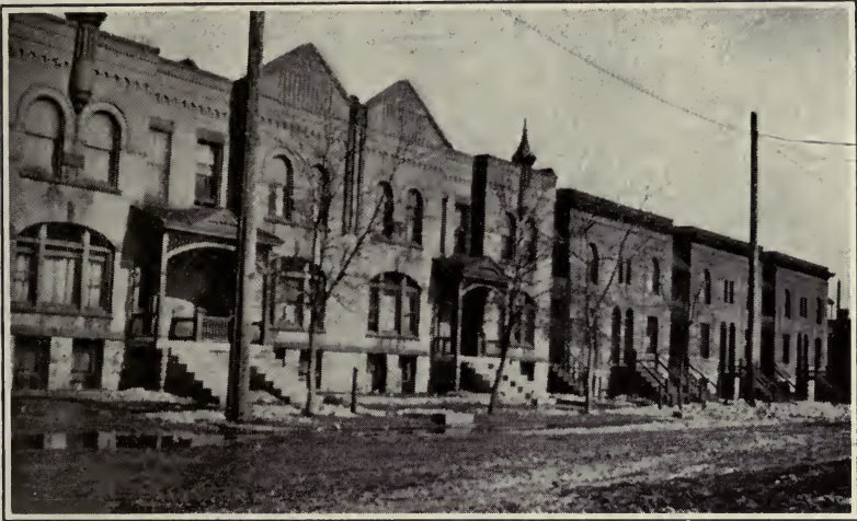
No. 11. Flats with dark room basements. Two buildings contain 46 dark rooms, 23 in basement apartments. In further building were old-fashioned long hopper closets, situated in basement and each used by three families.
