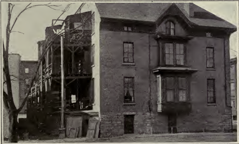
No. 12. Building has 23 apartments, each with dark toilet ventilating into living room. Sixteen apartments have from one to four dark rooms. Six garbage chutes, smeared their entire length with filth, add another unwholesome feature to the environment.
