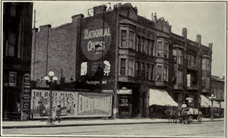
No. 17. Windowless wall. Apartments lighted only by windows in front and rear. Buildings contain 25 dark rooms.
