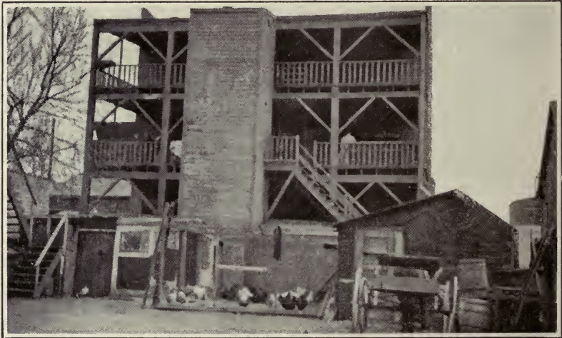
No. 31. Three-decker tenement privy and no yard.
