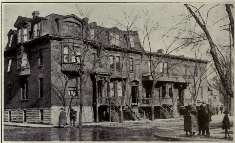
No. 13. Basement apartments said to flood during severe rains.
