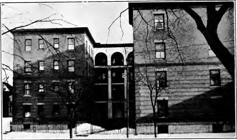
No. 23. Bathroom and kitchenette located in the same compartment is a "feature" of this apartment house. The bathroom ventilates over a dwarf partition and out through the kitchenette.
