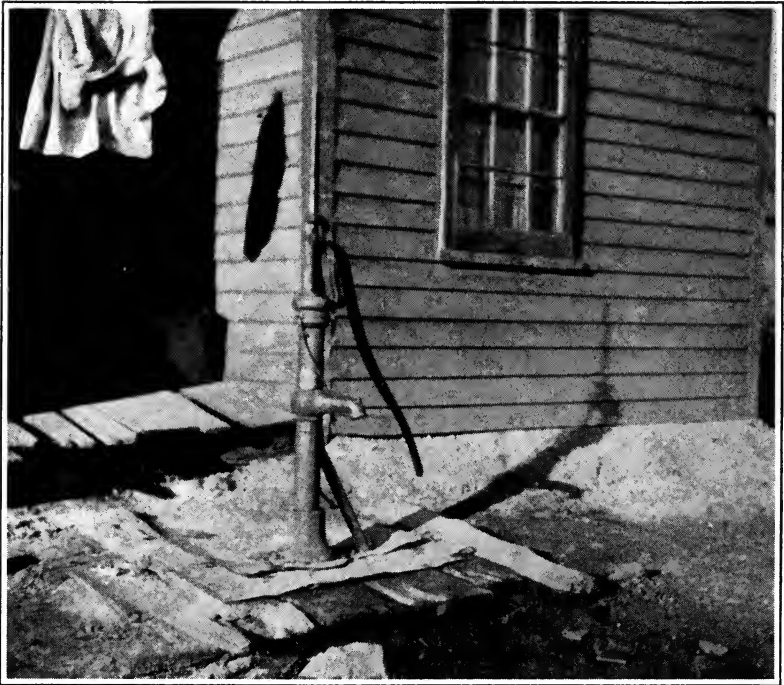
No. 47. An old well, the source of water supply for several families and the children of the neighborhood. Note the disk near the spout—shown more clearly in next illustration.
