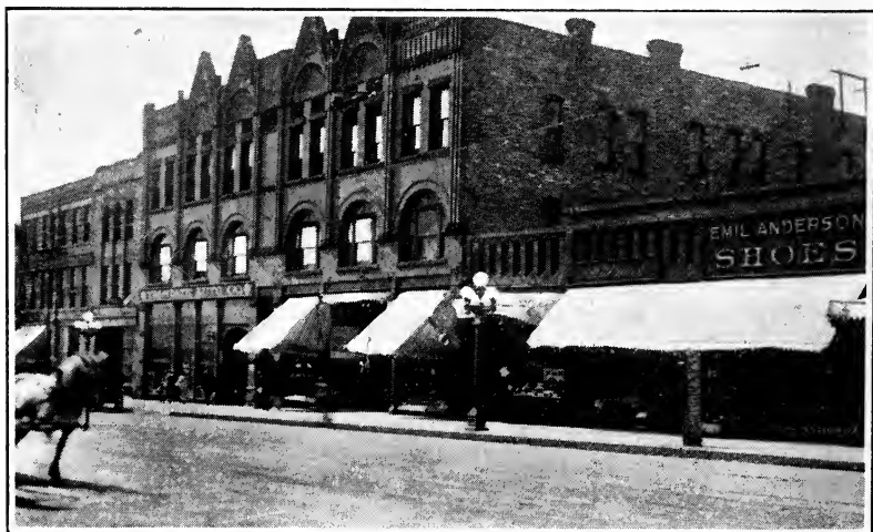
No. 19. How dark rooms are often made. Rooms lighted by windows in lot line wall become dark rooms when adjoining property is developed. Process complete on one side.
