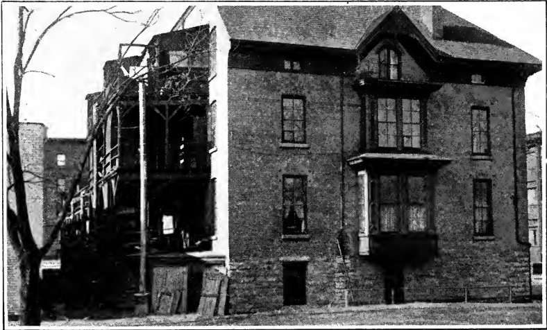
No. 12. Building has 23 apartments, each with dark toilet ventilating into living room. Sixteen apartments have from one to four dark rooms. Six garbage chutes, smeared their entire length with filth, add another unwholesome feature to the environment.
