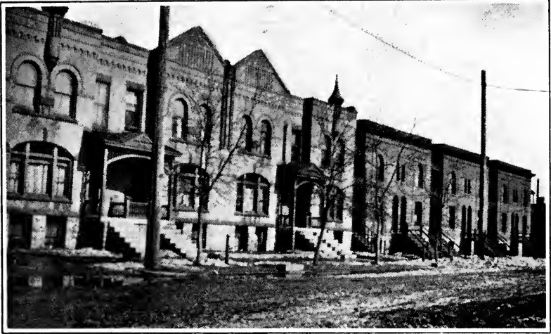
No. 11. Flats with dark room basements. Two buildings contain 46 dark rooms, 23 in basement apartments. In further building were old-fashioned long hopper closets, situated in basement and each used by three families.
