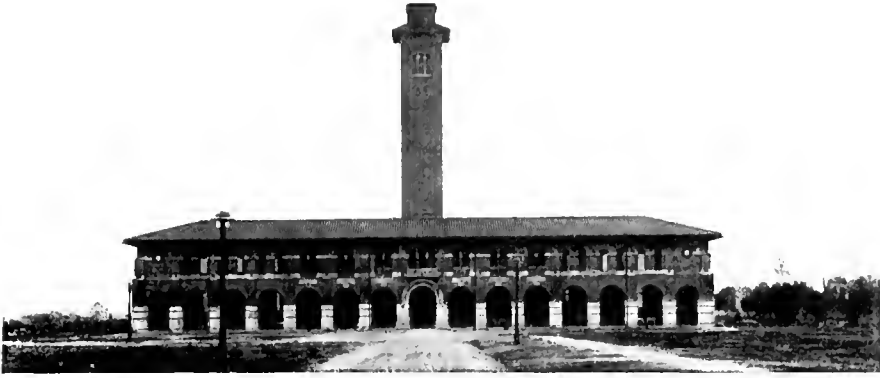
Mechanical Laboratory and Campanile of Power House
