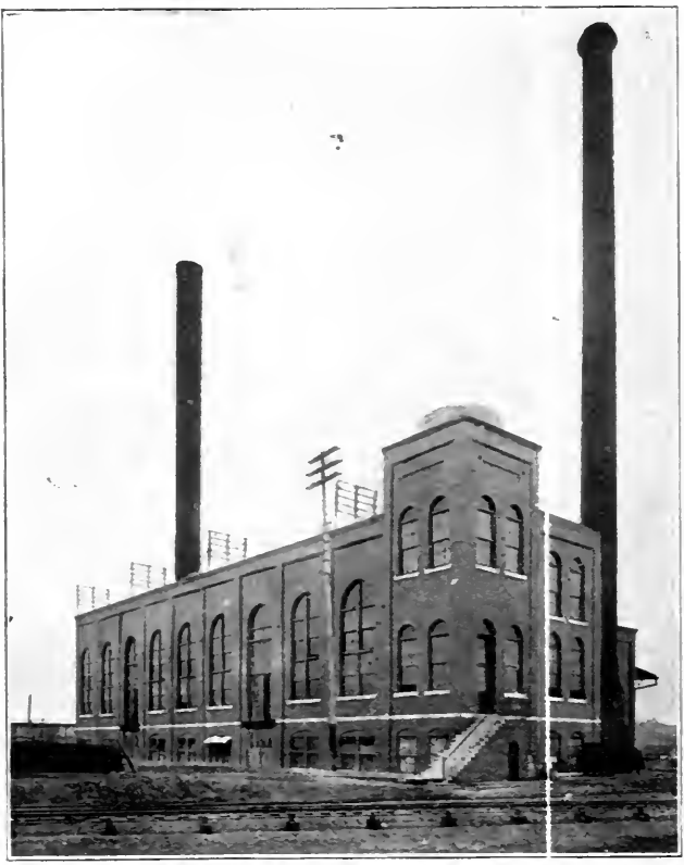
Electric Light and Power Plant
