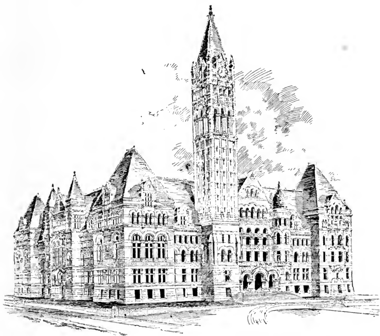
CITY AND COUNTY BUILDINGS (UNDER CONSTRUCTION), TORONTO.
