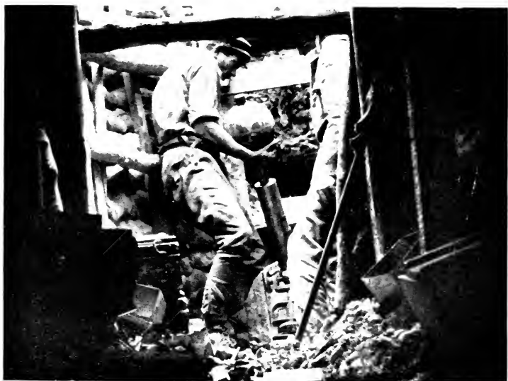
IN A TRENCH MORTAR TUNNEL, DURING THE BATTLE OF THE SOMME, AT BEAUMONT HAMEL, JULY 1ST, 1916
