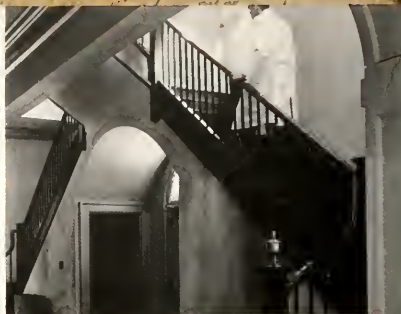
Stairway above entrance to Medical Building.
