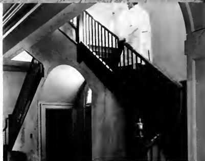
Stairway above entrance to Medical Building.
