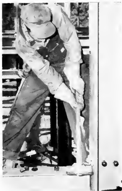
Working on the New Wing.
