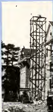
One of the new buildings illustrative of the construction work.
