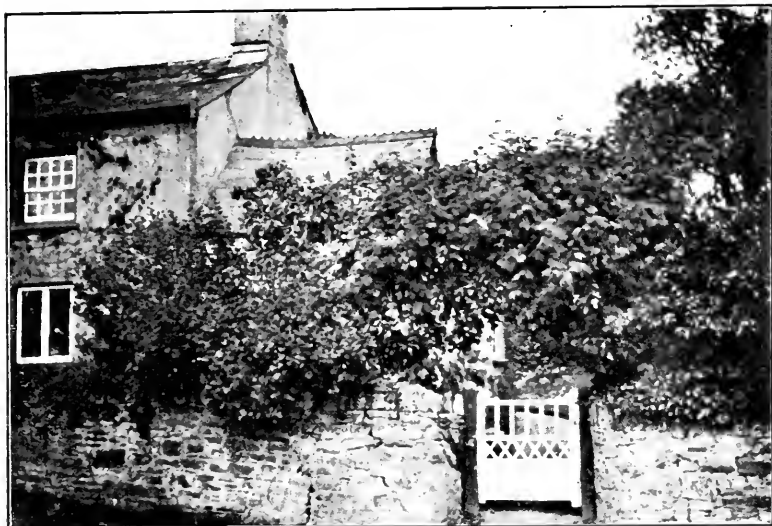
PLATE XXIII. Wall and gate to kitchen entrance. Note good design for gate and poor bonding in construction of wall.
