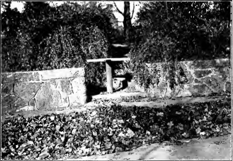
PLATE XIV. Well built wall, note raked out joints and slight batter. Turnstile instead of gate.
