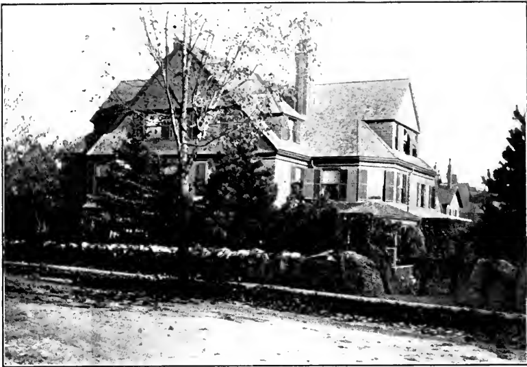
PLATE XVII. Wall built of boulders and ledge stone covered with vines. Top of stones are about three feet above sidewalk.
