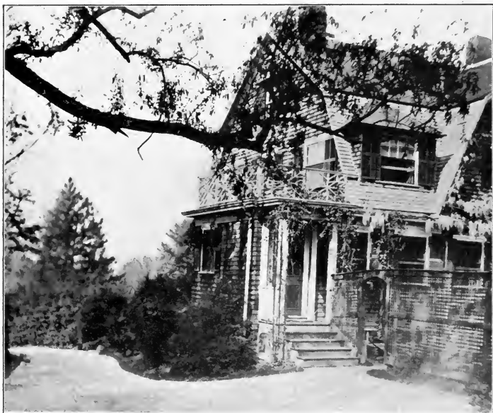
PLATE X. Drive located on simple curves at side of property, carriage turn close to kitchen door and laundry yard. Visitors alight halfway up the drive. Shrubbery border screens drive from house lawn.
