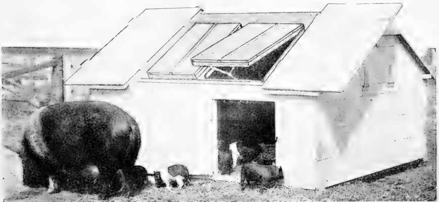
Fig. 18—Individual Hog House with Sunlite Windows.
