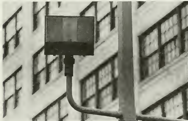
New high-efficiency sodium light replaces old light on this parking lot pole.
