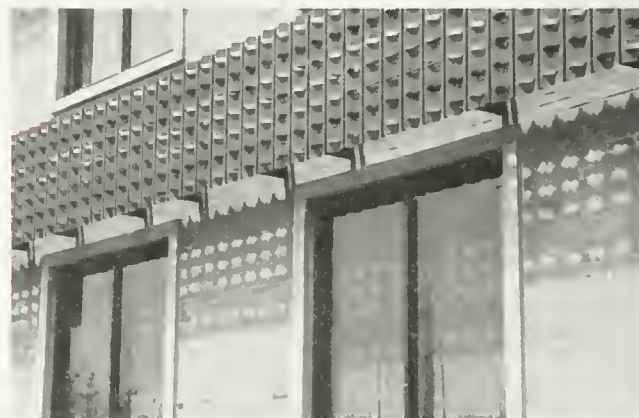
On high school converted to office building, lattices provide horizontal design accent and shield windows from sun's heat.
