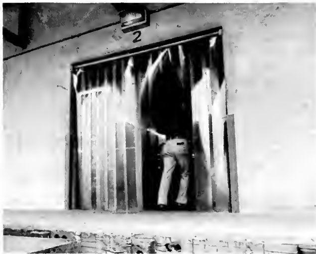
Curtain of plastic strips made by wholesale company's owners is used year round, prevents both heat loss and gain while permitting access to loading dock.
