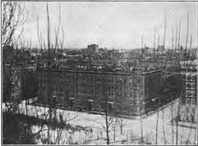
FIG. 7. — An Apartment House in New York City.
