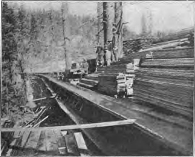
FIG. 43.—Boards ready to be Flumed.
