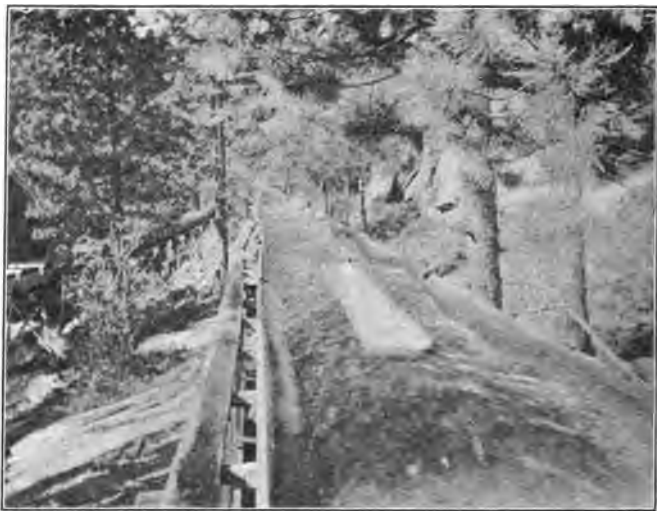
FIG. 44. — Boards going down a Flume.
