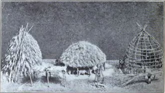
FIG. 15. — Wichita Indians building a House.
