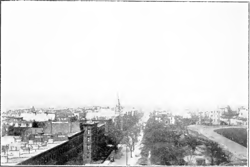
VIEW OF HUDSON STREET AND PORTION OF STEVENS CAMPUS
