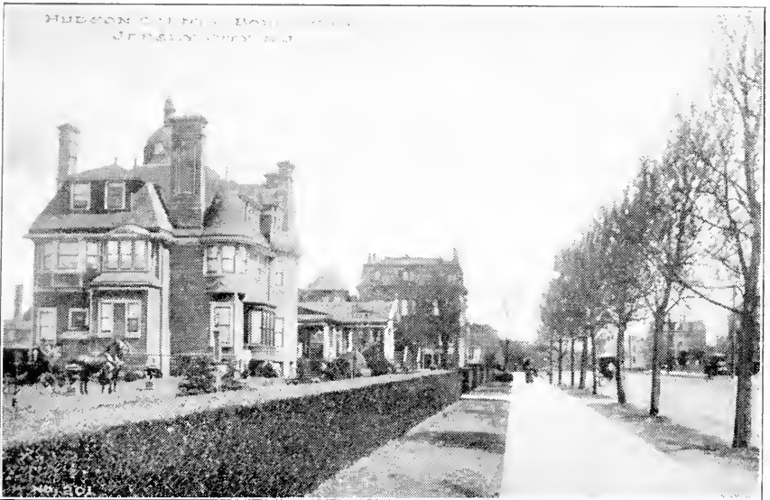
HUDSON COUNTY BOULEVARD, JERSEY CITY, N. J.
