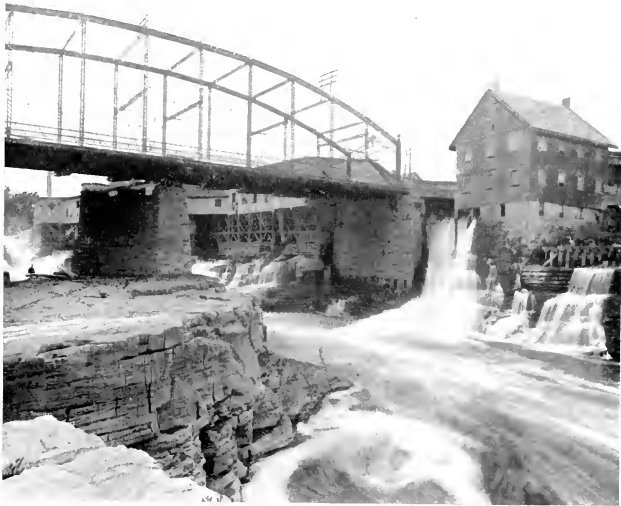
THE BRIDGE AT GLENS FALLS
