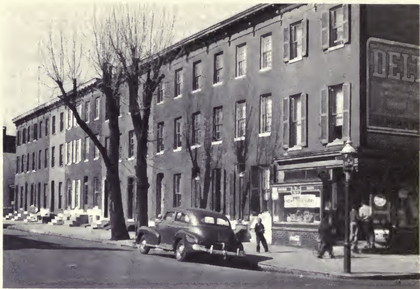
A typical block of Pilot Area homes. This is the 1700 block of East Chase Street. The confectionery on the corner is also typical of the scattered commercial properties in residential blocks.
