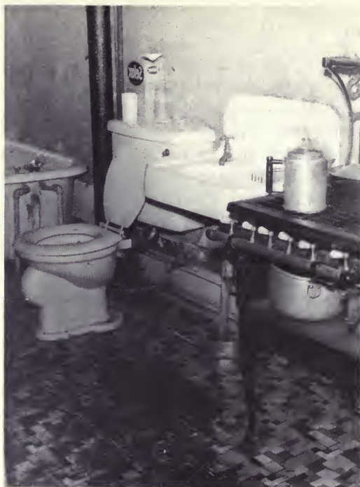
A Mount Royal space-saver: same room doubles as kitchen and bath in a single-family home converted to apartments. This sort of health code violation was stamped out by the law enforcement program, although the exterior of the building showed no change.
