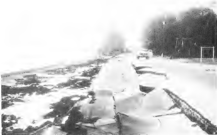
Photo 12. Highway damage near Carrabelle, Fla.
