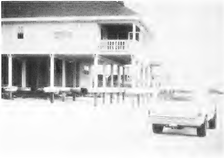
Photo 8. Beach erosion under house, Cape San Blas, Fla.
