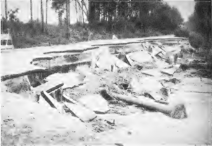
Photo 11. Highway damage between Cape San Blas and Carrabelle, Fla.
