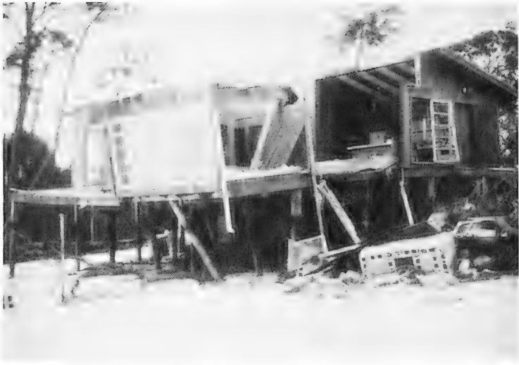
Photo 15. House destruction between East Point and Carrabelle, Fla.
