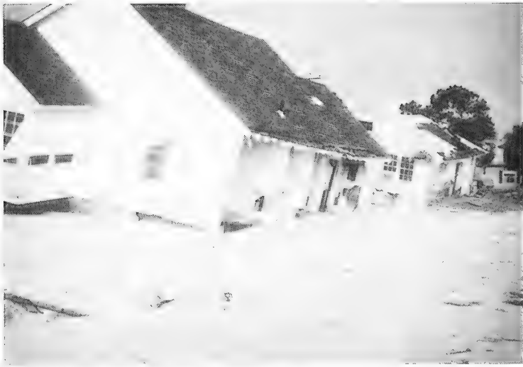
Photo 16. House destruction, Lighthouse Point, Fla.
