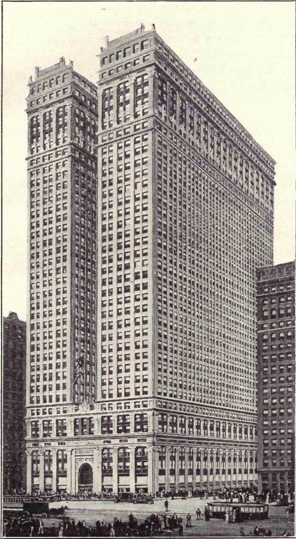
EQUITABLE BUILDING, NEW YORK CITY R. E. GRAHAM, CHICAGO, ARCHITECT Hydrated Lime Used Throughout in All Brick Mortar
