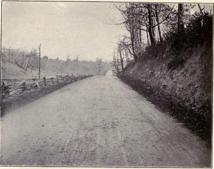
CONCRETE ROAD, GARRET CO., MARYLAND 10% Addition of Hydrated Lime to 1-2-4 Concrete (Monolithic Type)
